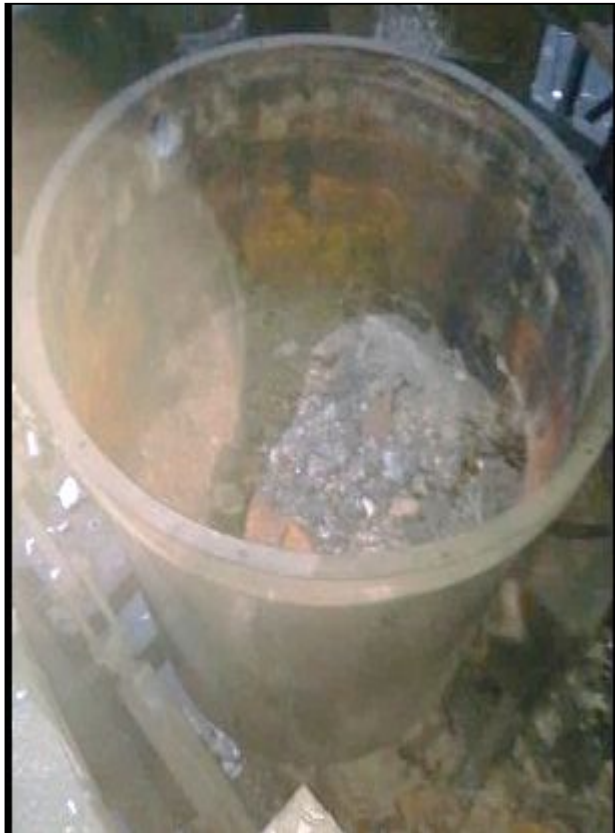
Furnace shell cleaned & Initial HR Paint removed
