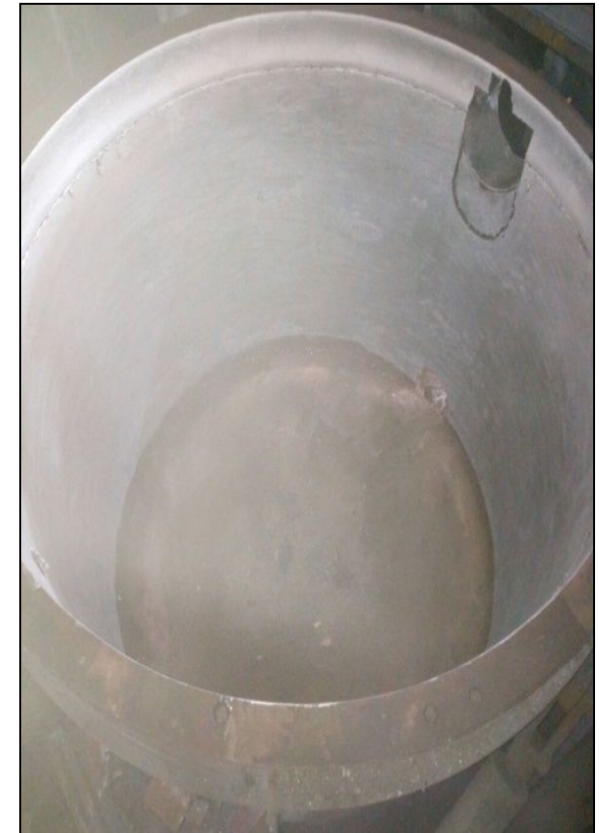
Inside Surface Coated with HRTI-400
